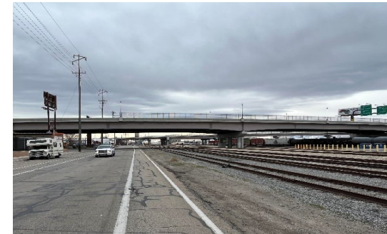
Figure 18. UPRR at 600 West in the Granary District
